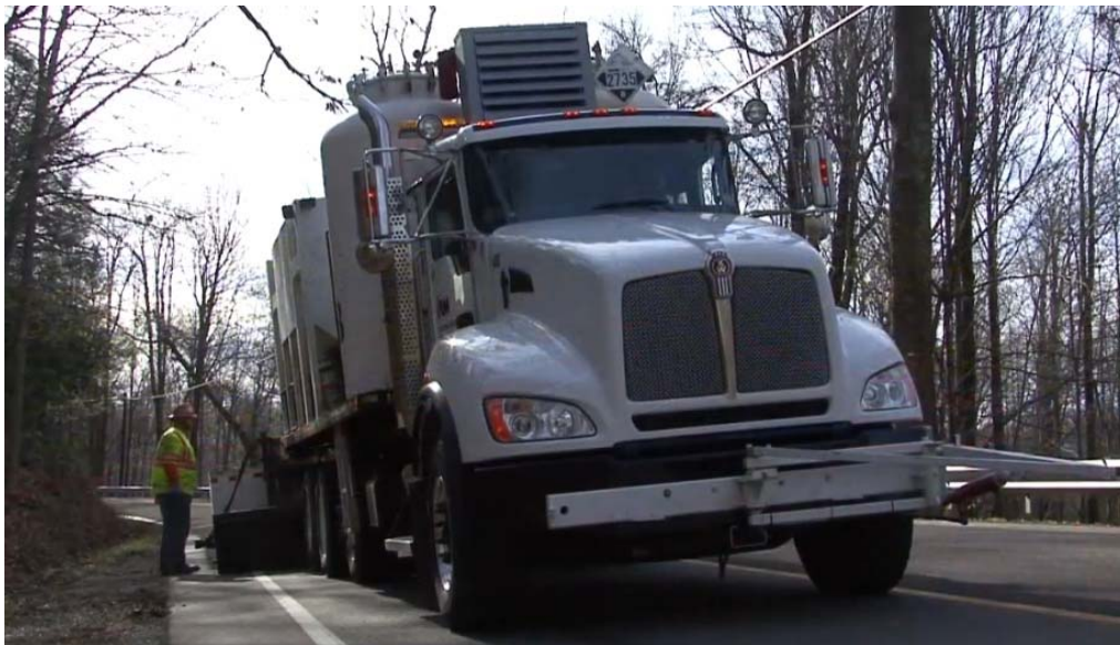
Figure 5: Application of an HFST by truck.
