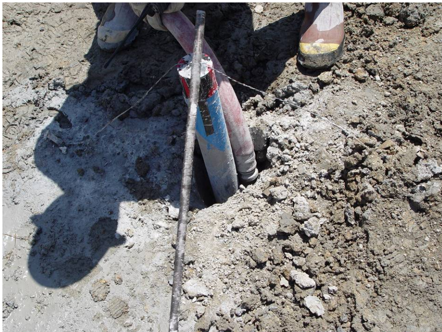
Figure 5.27 Field schematic of inclinometer anchoring and grouting.
