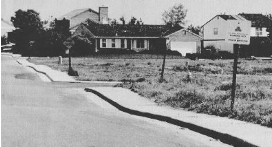
Figure 2.3 Pavement overlying expansive soils and subjected to distress due to shrink-swell movements. (Source: www.surevoid.com ).
