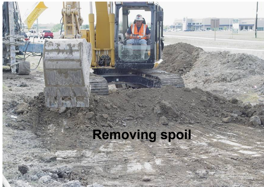
Figure 5.18 Removal of spoil from the surface at end of DSM treatment.
