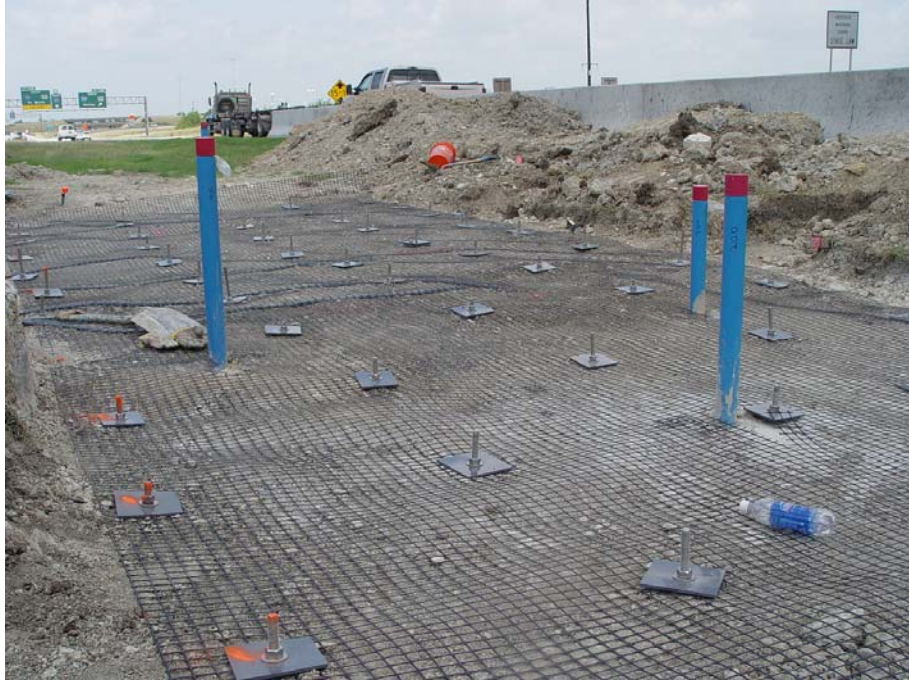
Figure 5.19 Test section after fastening geogrid to DSM columns using anchor rod and plate-bolt system.
