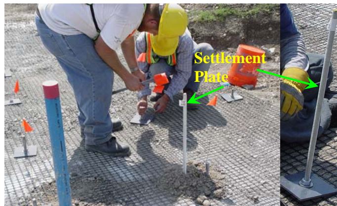
Figure 5.34 Settlement plate and its placement.
