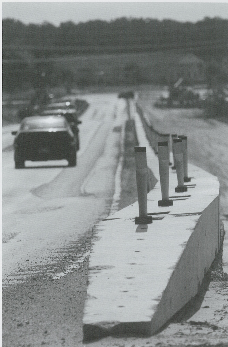
A very simple licensing process will now allow other states to use the low-profile portable concrete barriers developed at TTI.
