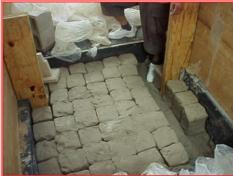
FIG 3 Preparation of the Clay Soil Tank
