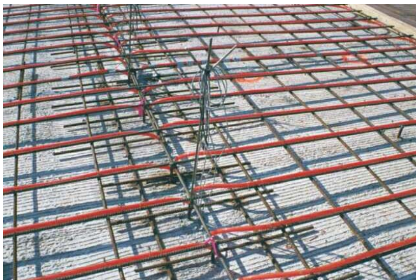
Figure 13-6. Bridge Deck Showing Instrument Wire on Trees.
